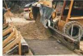
Installation Damage
