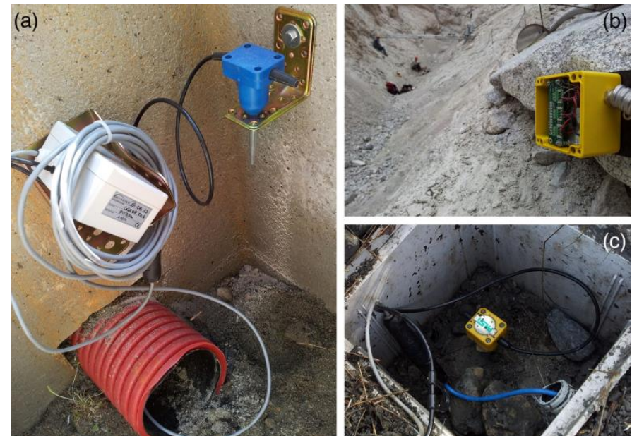
Geophone installation methods: (a) embedded in concrete, (b) fixed on rock surface; (c) dug in the ground (Coviello, 2015)
